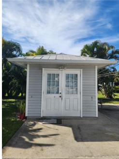
Front of Shed
